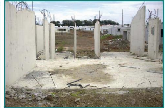
Figure 3: Finished concrete walls
