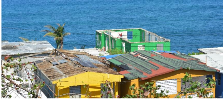
Collateral wind damage to properties in Old San Juan, Puerto Rico
