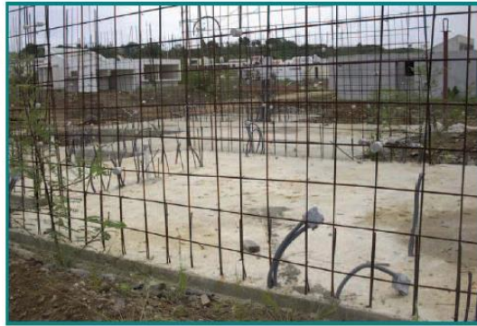
Figure 2: Steel Reinforcement
