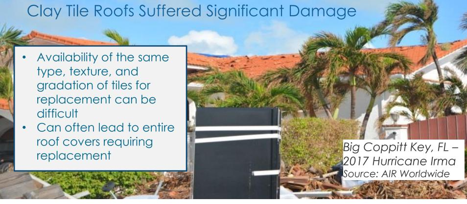
Mortar and adhesive-set clay tiles suffered the most damage in comparison to mechanically attached ones
