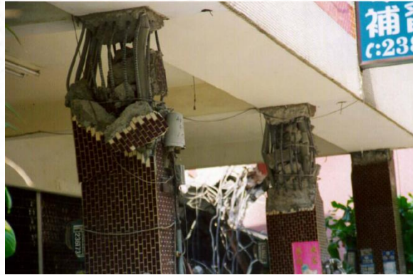
Reinforced Concrete Building Damage: Model vs. Observation in Chi-Chi Earthquake
