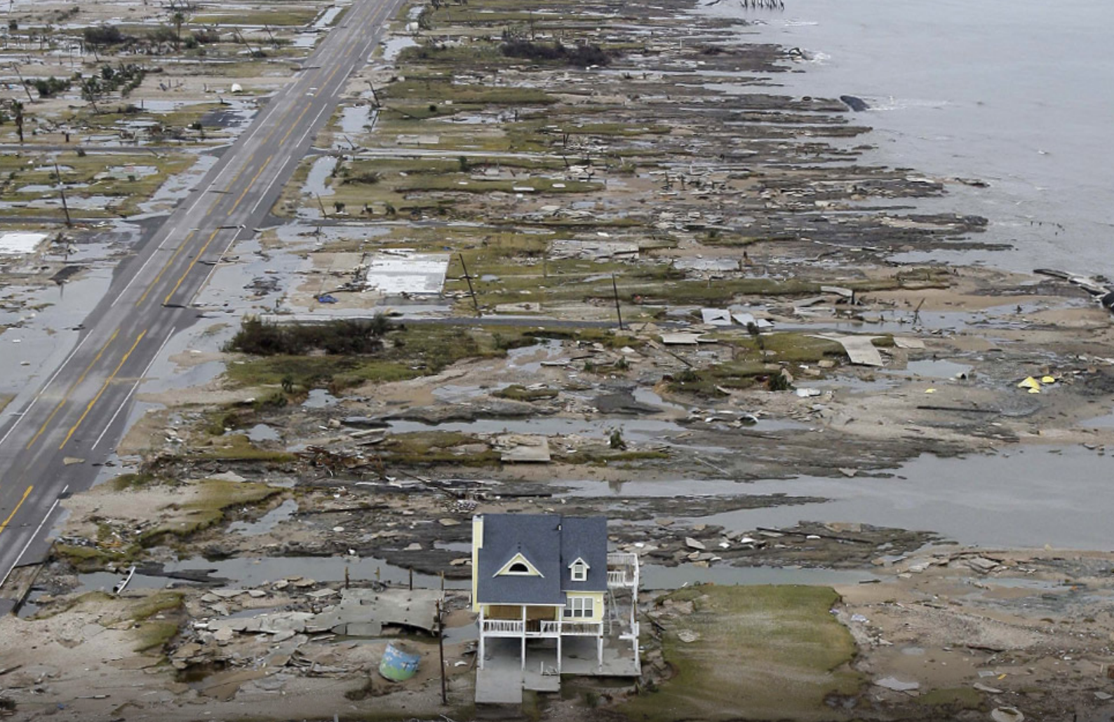
Hurricane Ike storm surge devastation of Bolivar Peninsula near Galveston, Texas. (Source: Chuck Davis, flickr)
