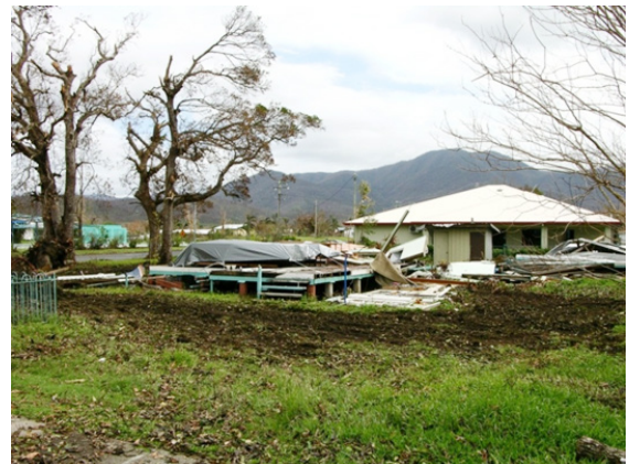
In Australia, building age is an important factor in determining building vulnerability. Here, a newer building in Cardwell was left standing by 2011's Cyclone Yasi, while an older one beside it was destroyed. (Source: AIR)
