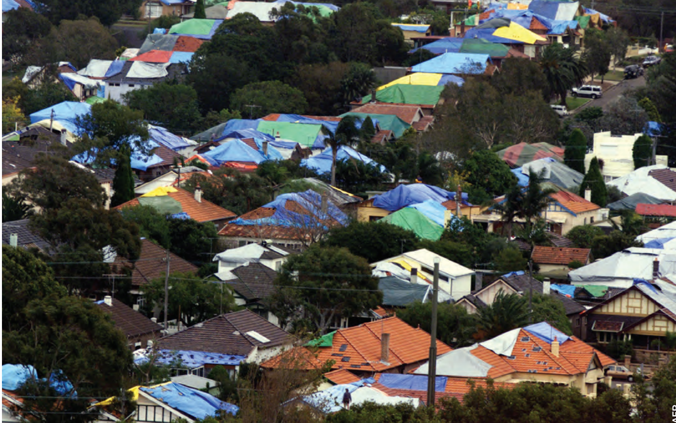
Costly catastrophe: damage following Sydney's 1999 hailstorm
