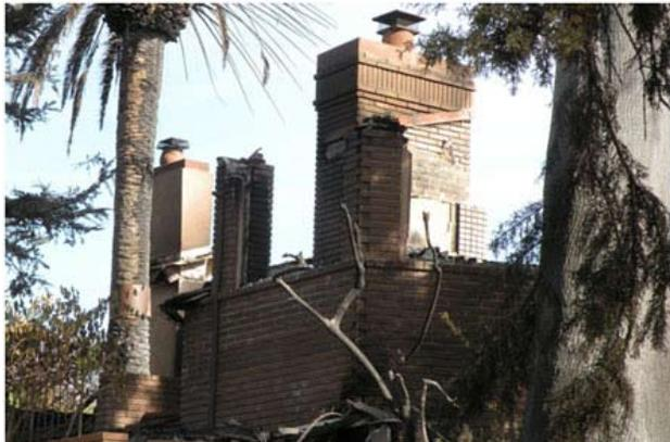
Figure 6. Masonry survives even when nothing else does. Source: AIR
