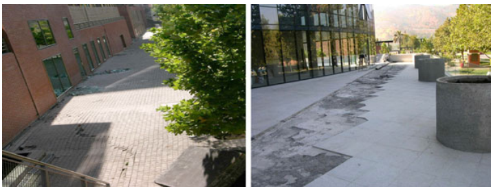
Figure 9. Settlement (left) was observed outside buildings in La Ciudad Empresarial. Cracks (right) propagated along the ground due to soil settlement. (Source: AIR).
