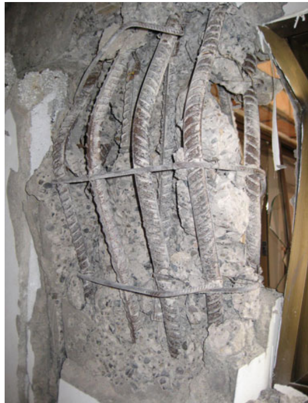
Figure 11. Buckled longitudinal rebar in structural wall of Viña del Mar building (Source: AIR).
