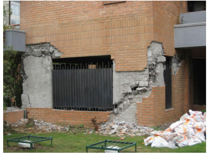
Figure 10. Partial collapse of high-rise apartment building in Viña del Mar. (Source: AIR)
