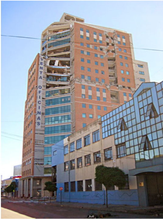
Figure 5. The Torre O'Higgins high-rise suffered severe damage and is scheduled for demolition. (Source: AIR).
