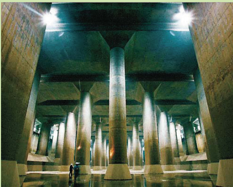
Figure 1: Example of an underground cistern located north of Tokyo. Note the relative size of the people (Source: Yomiuri Shimbun).
