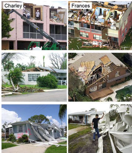
Figure 2. Despite their vastly different wind speeds, damage patterns near the landfall locations of fast-moving Hurricane Charley (left column) and slow-moving Hurricane Frances (right column) were remarkably similar. (Source: AIR and Various)
