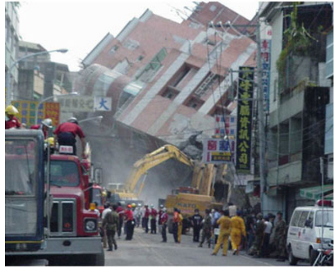
Figure 2. Toppled Building in Chi-Chi (Source: AIR)
