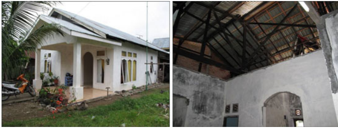
Figure 3: Residential house in Padang (left) and typical roof configuration (right). (Source: AIR)
