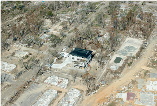
Figure 2 .This mitigated home in Long Beach, Mississippi, survived Hurricane Katrina when its neighbors did not (Source: FEMA/Mark Wolfe)
