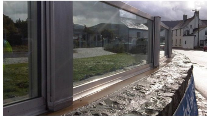
Figure4. A glass wall flood defense in Keswick, Cumbria (Source: ITV)
