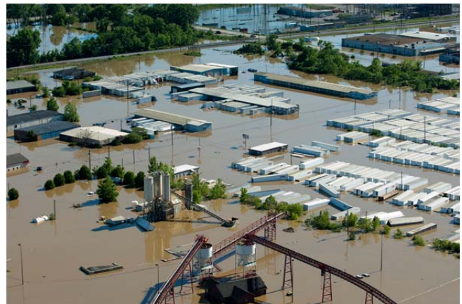
The 2010 Cumberland River flood, Nashville, Tennessee. (Source: FEMA)
