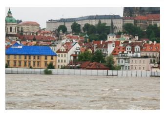
Record-breaking flooding across Central Europe in 2013 caused significant insured losses. Flood defenses like this dike on the River Vltava (Moldau) in Prague—constructed during the 2013 flood event—are built in advance of flooding to protect against rising water. AIR's Inland Flood Model for Central Europe accounts for the impacts of levees, dikes, and flood walls, as well as mobile and temporary defense barriers.
