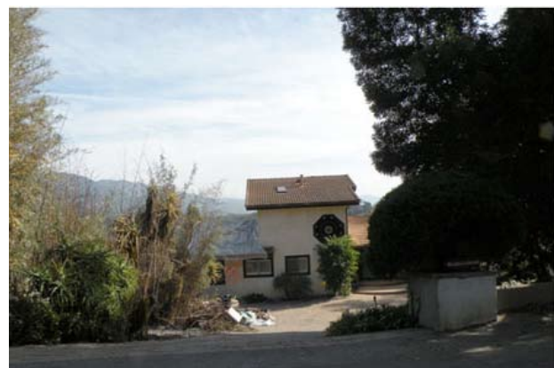
Figure 5. One of the rare cases of “partial” damage. Source: AIR
