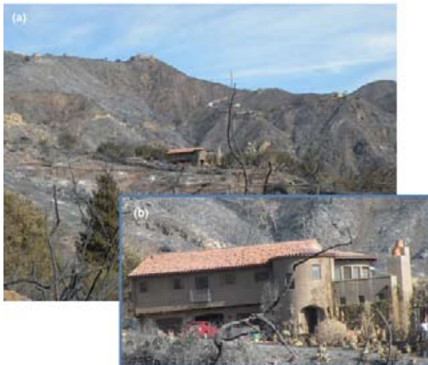
Figure 7a and b (inset). Surroundings completely burned, but brush setbacks and good construction won this particular battle. Source: AIR
