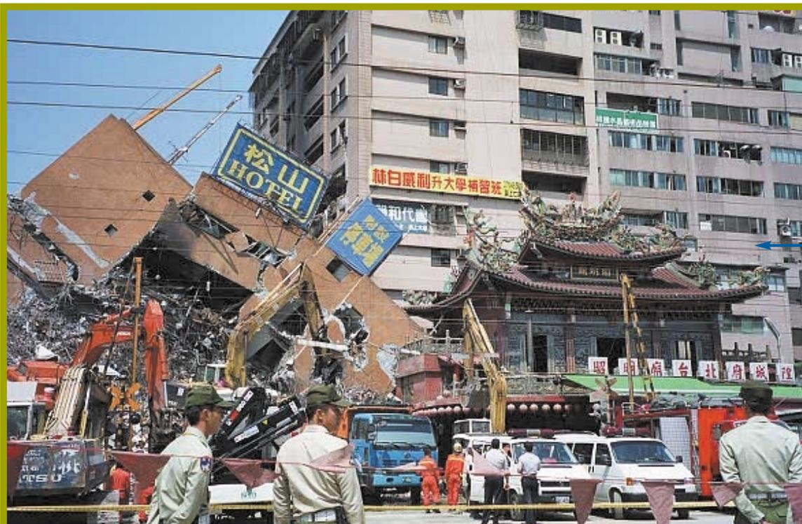
*The spottiness of damage was strikingly evident in both the Ji-Ji and Izmit earthquakes. In this photograph, one modern building has completely collapsed, while others remain intact, including an old temple built without the benefit of seismic design.*
