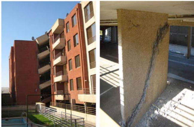
This building in Maipú, greater Santiago, partially collapsed due to shear wall failure caused by the 2010 Maule quake. (Source: AIR)
