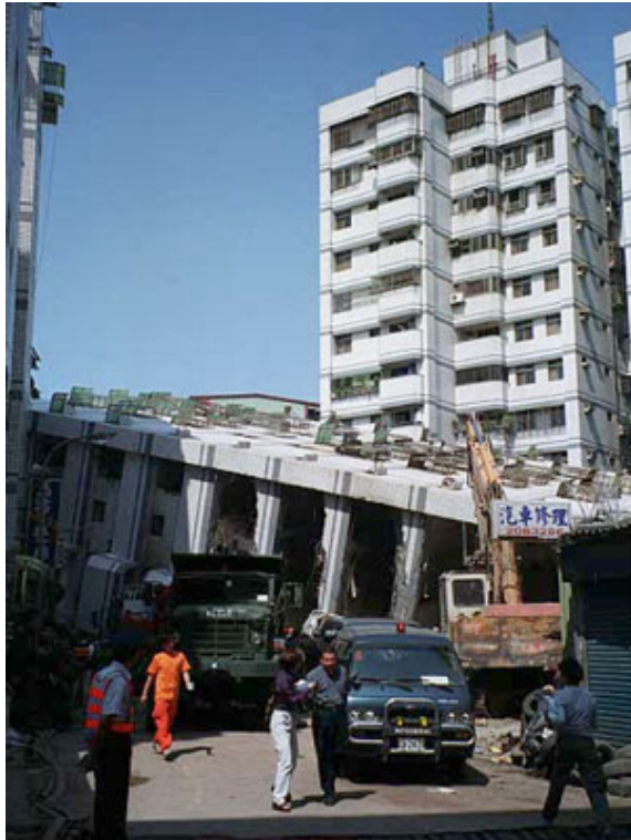
Figure 2. During the 1999 earthquake in Chi-Chi, Taiwan, one apartment building toppled to the ground, while an identical one nearby remained intact, illustrating the need to account for aleatory uncertainty (Source: AIR)
