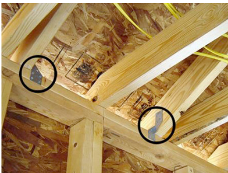
Figure 1. Clips help anchor roofs to the main structure to prevent detachment due to severe wind (Source: FEMA/Yonah Walter)
